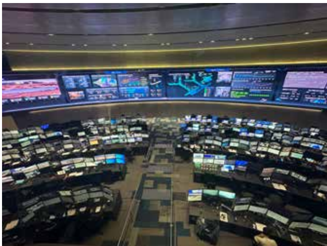
AVSECO's massive control room
