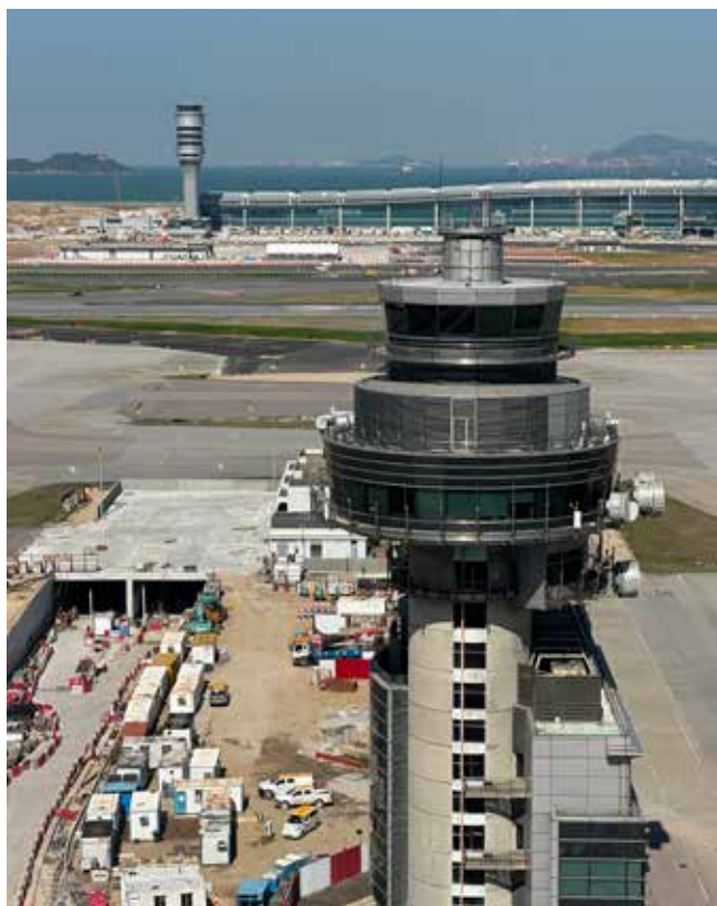
Two of Hong Kong Airport's three towers
